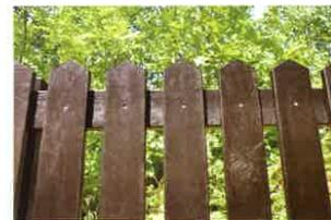
Plaswood high performance lumber is made from 100% recycled plastic and offers a no maintenance solution: unlike conventional wooden decking or lumber (aka timber), Plaswood doesn't require annual maintenance, staining or painting.
