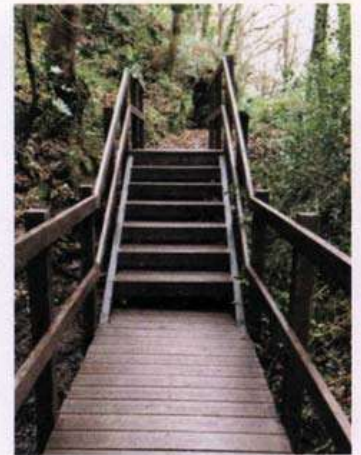
New Plaswood stairway, made from 100% recycled plastic
