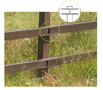
Posts can be anchored to the ground using the same method as timber and steel posts, by concreting, hammered mechanically or surface fixed.
